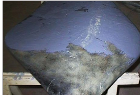
Use fiberglass mesh as reinforcement
